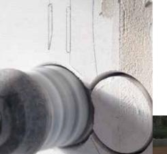
AAC product densities vary between 300 - 800kg/m³ and compressive strengths are between 2,5 - 7 N/mm². The finished product volume is 3x the volume of the raw materials used, making it an extremely resource-efficient and environmental friendly building material.
