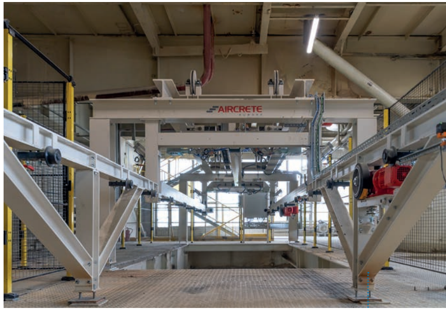
Storage area, the so-called buffer
